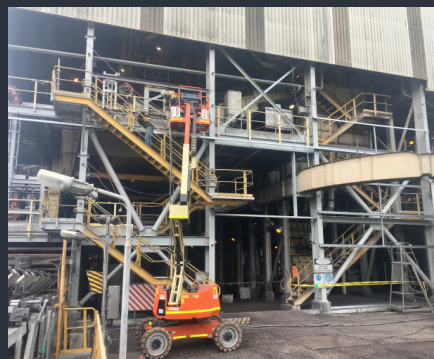
CHPP Structural Steel Painting
