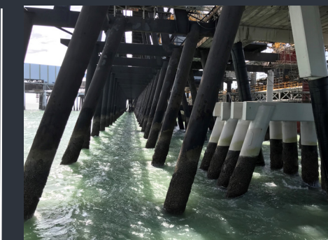
Jetty Pylons & Headstocks
